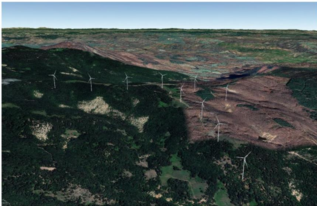
Picture 13: Panoramic view of the WPP with shooting direction north.
