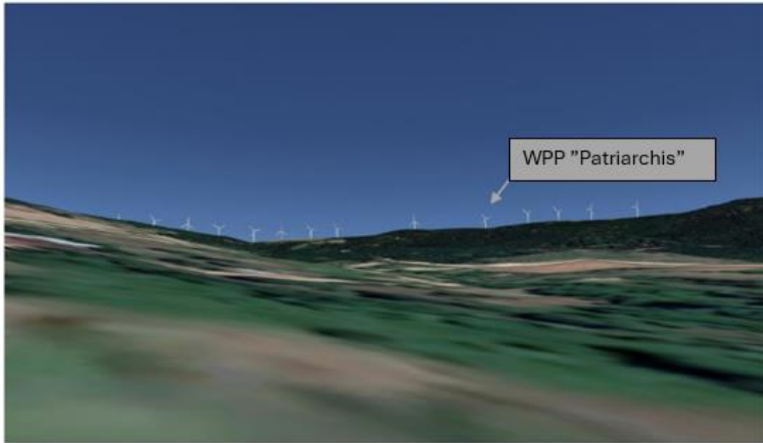
Picture 8: View of the WPP from the "Chloi" village.
